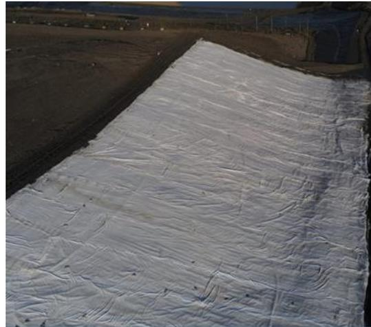
Soils have been stockpiled in readiness to be placed on the HDPE plastic cap; currently hindered with the serve weather.
